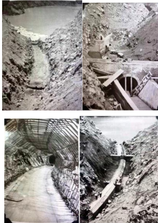
New tunnel being constructed in the early 1980s. First the channel was cut, then the tunnel built, and finally the canal was covered with a safety dam. Photos: César Portocarrero
